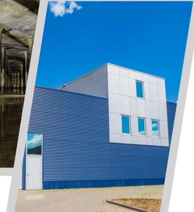
WATER PUMPING STATION
