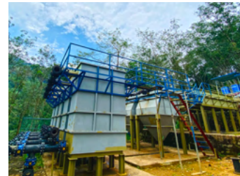
Construction of Bulathkohupitiya Integrated Rural Water Supply Scheme 1000m 3 /day Package Treatment Plant
