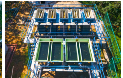
Construction of Bulathkohupitiya Integrated Rural Water Supply Scheme 1000m 3 /day Package Treatment Plant
