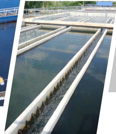
RAPID SAND FILTER & GAC FILTERS
