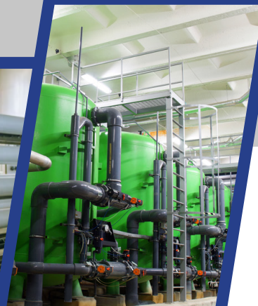
DE-MINERALIZATION PLANT
