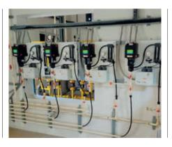
of-the-art GAS Chlorination System to disinfect the water supply. The system will inject controlled streams of chlorine solution to treat the water supply and will maintain residual chlorine in the distribution system to ensure safe drinking water at consumer outlets. This Gas Chlorination system supplied and installed by DIMO is fully automatically controlled and is capable of effectively catering to the demands received from the Supervisory Control & Data Acquisition (SCADA) system.
