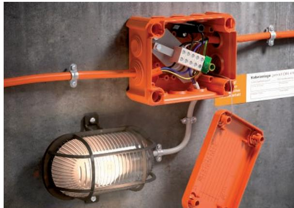
Junction boxes which have the capability to maintain electrical function ensure the fireproof connection of the safety cables. The boxes in the FireBox series are tested and approved to maintain electrical function for 30 to 90 minutes in accordance with DIN 4102-12.
