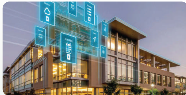
Building Services - Lighting, Elevators and Escalators, Extra Low Voltage (ELV)
