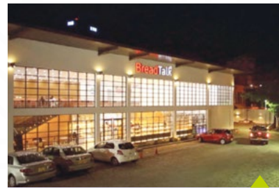
RIL Building, RIL Properties (Pvt) Ltd, Colombo 2
