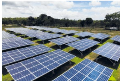
IMW Ground Mounted Solar PV System, Embilipitiya
