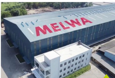
WMR Project, Melwire Rolling (Pvt) Ltd
